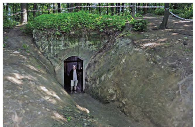
The recently excavated entrance to the Kamzik bunker
